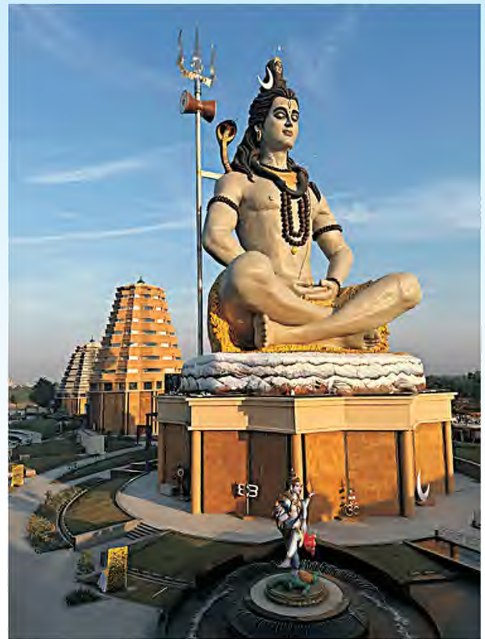
After Construction (Shiv Dham) Char Dham, Vrindavan (U.P.)
